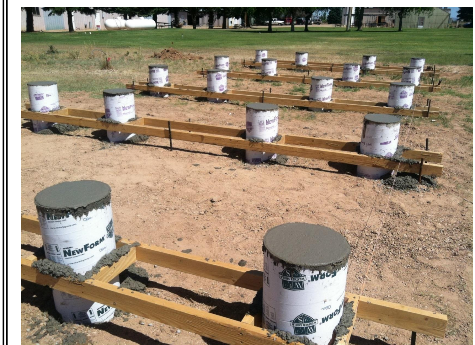
Fig. 4. Concrete piers for foundation
