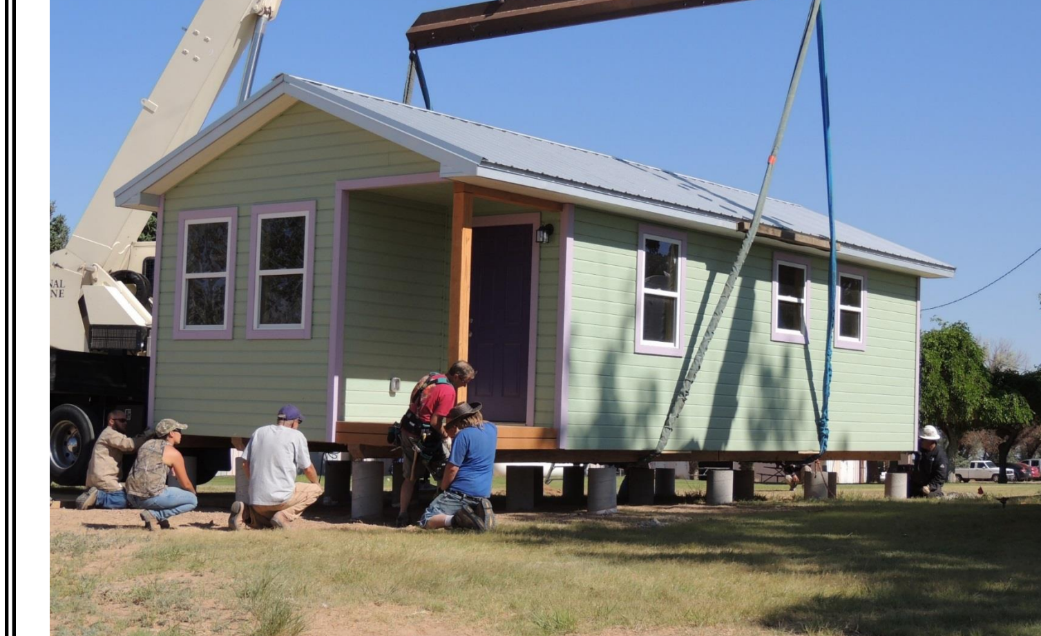
Fig. 5. Transporting the house from SJC campus to NMSU-ASC Farmington permanent location
