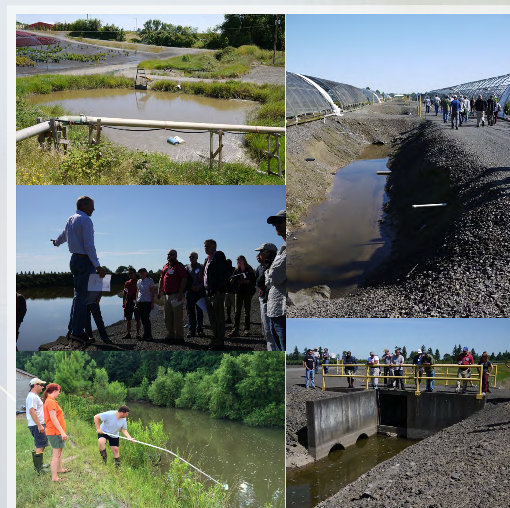
Figure 6. Water conveyance structures and Clean Water 3 team monitoring and evaluation of site challenges.
