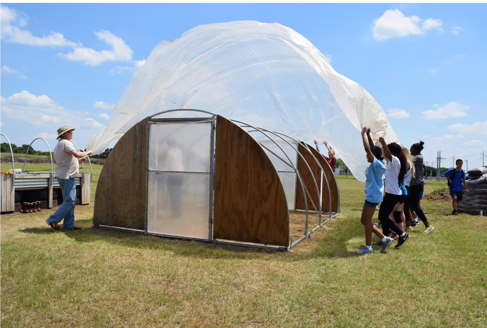
Photo 5: Constructing a hoop house at Noble Research Institute, Ardmore, OK
